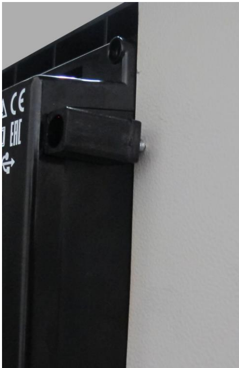
Installation of screw type bracket
