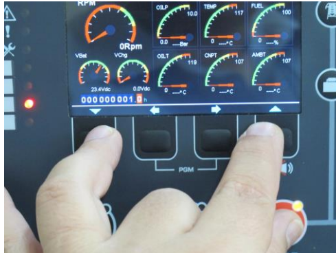
Hold pressed OFF, LAMP TEST and ALARM MUTE
