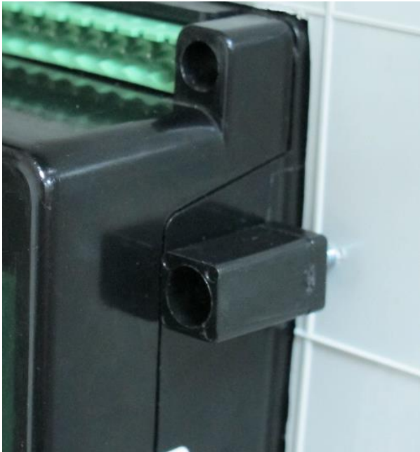
Installation of screw type bracket
